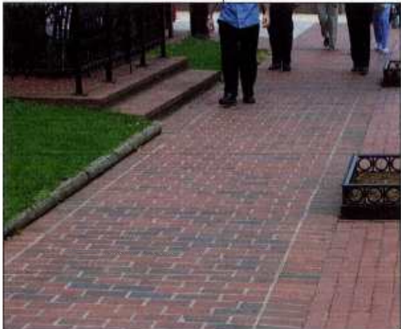
Exhibit 3-13. Brick Sidewalk. Photo courtesy of James T. McDonnell.
