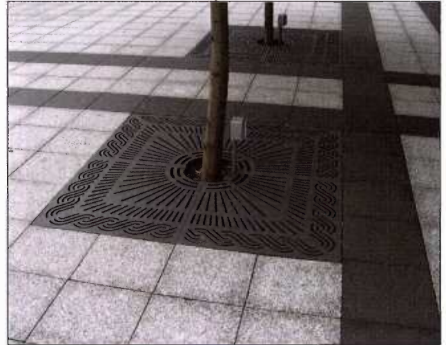
Exhibit 3-16. Well-Designed Sidewalk Tree Grate.
